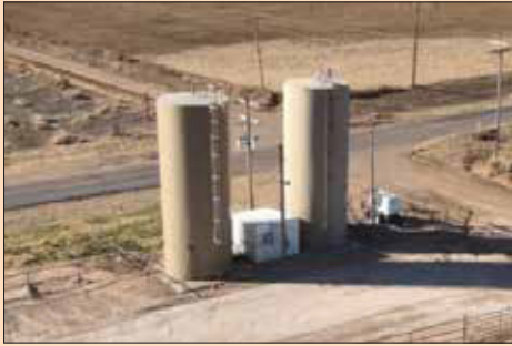
30,000 Gallon Water Storage Tanks
