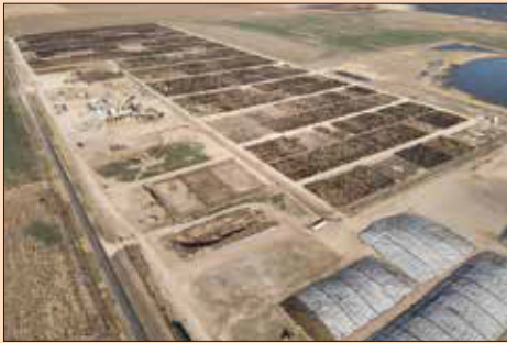
SE Yard Overview
