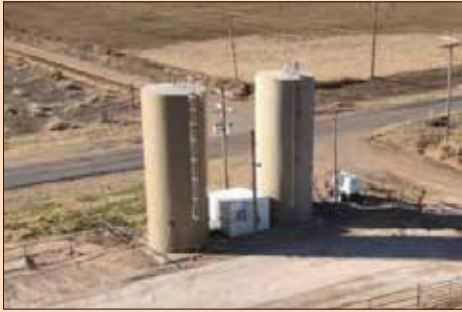
30,000 Gallon Water Storage Tanks
